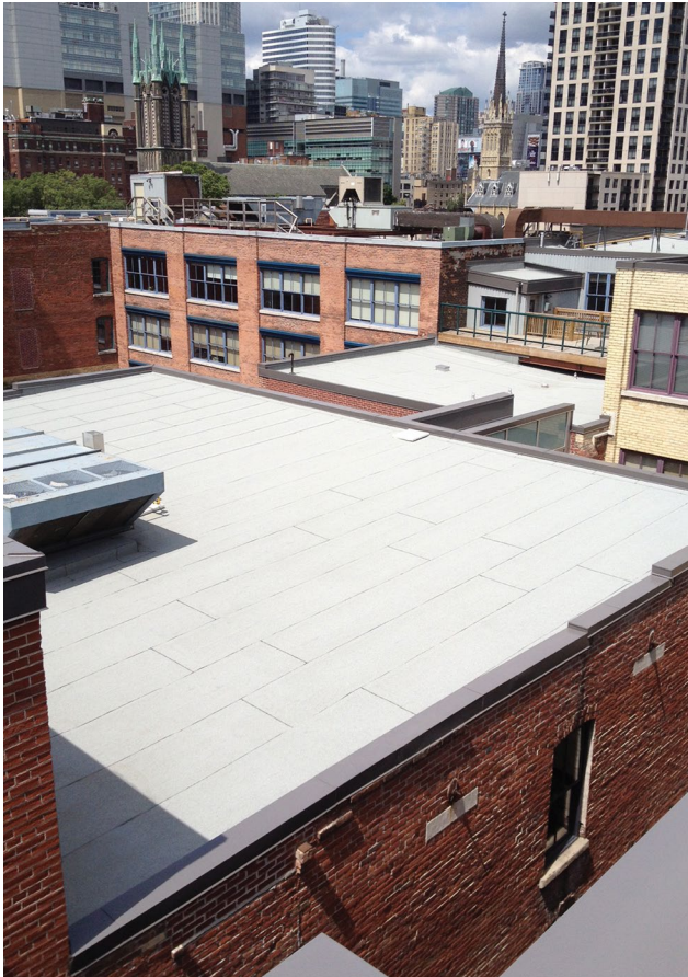
Low-slope roofing membrane with self-adhered SBS base sheet and torch-applied SBS sheet.
