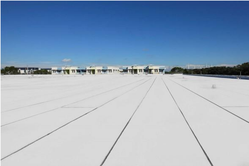
Low-slope roofing membrane with self-adhered SBS base sheet and torch-applied SBS cap sheet.
