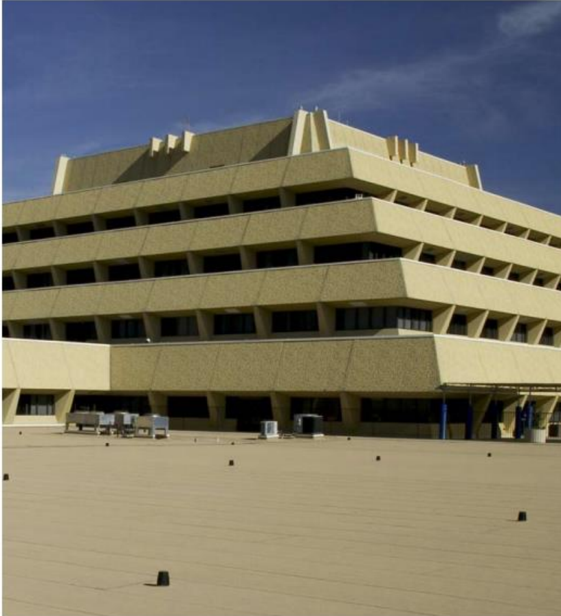
Low-slope roofing membrane installed using hot asphalt and consisting of a SBS-modified bitumen cap sheet and a SBS base sheet.
