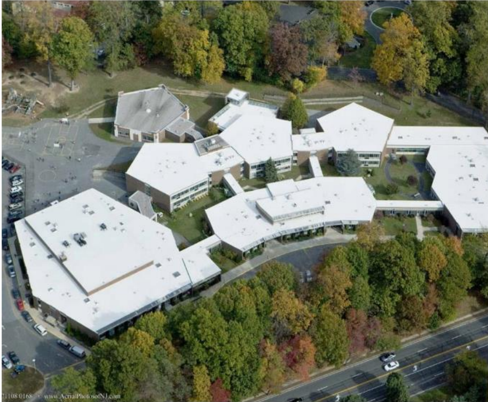
Low-slope roofing membrane installed using low-VOC adhesive and consisting of a modified bitumen cap sheet and base sheet.
