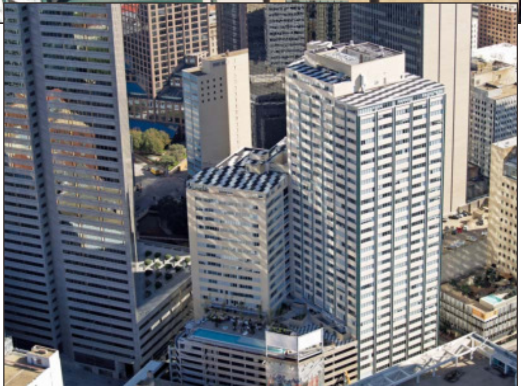
This downtown Dallas building was renovated into luxury condos. The developers wanted it to be seen by the high-rise buildings around it. Construction: Iso set in OlyBond 500, Liberty SA, SBS heat-weld 25, SBS heat-weld FR seen as white, Torch Plus FR seen as black.
