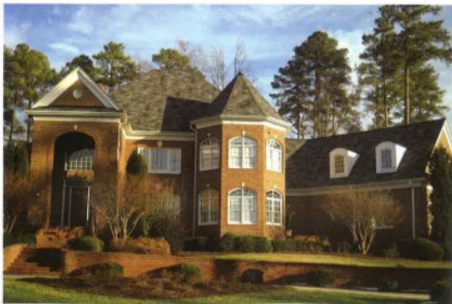
Photos courtesy of ASPHALT ROOFING MANUFACTURERS ASSOCIATION, Washington, D.C.
