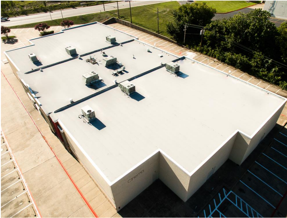
Low-slope roofing membrane installed using a propane torch and consisting of a SBS-modified bitumen cap sheet and base sheet.
