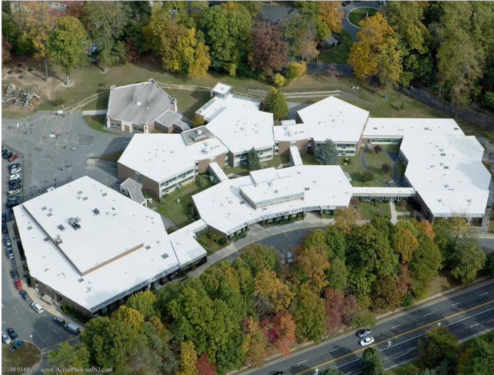
Low-slope roofing membrane installed using low-VOC adhesive and consisting of a SBS-modified bitumen cap sheet and base sheet.
