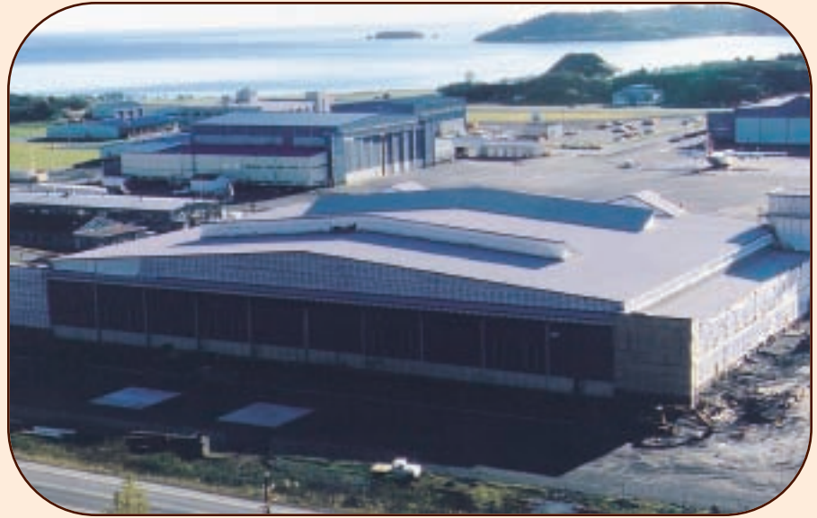
Winds of 50 mph to 100 mph are common at the Coast Guard Naval Air Station on Kodiak Island, Alaska. This facility was used to house fighter planes in the 1940s and now houses Coast Guard airplanes and helicopters. Two historic hangars with a total area of 1,480 squares are covered with a smooth-surfaced APP-modified bitumen roof membrane capped with a mineral-surfaced APP-modified bitumen cap sheet. The membranes were torch-applied. Photo courtesy of CertainTeed Corp., Valley Forge, Pa.
