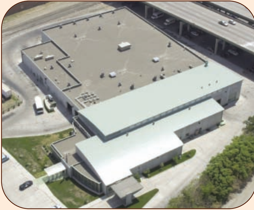
The Wichita Transit System facility houses buses and vans, as well as administrative offices. A gray color was used to enhance the appearance of the cap sheet because this facility is visible from a nearby highway that passes above it. Photo courtesy of CertainTeed Corp., Valley Forge, Pa.
