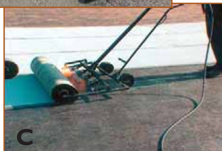
Asphalt roofing application methods include A) hot-applied, B) cold-applied, and C) torch-applied. (Photos courtesy of ARMA.)
